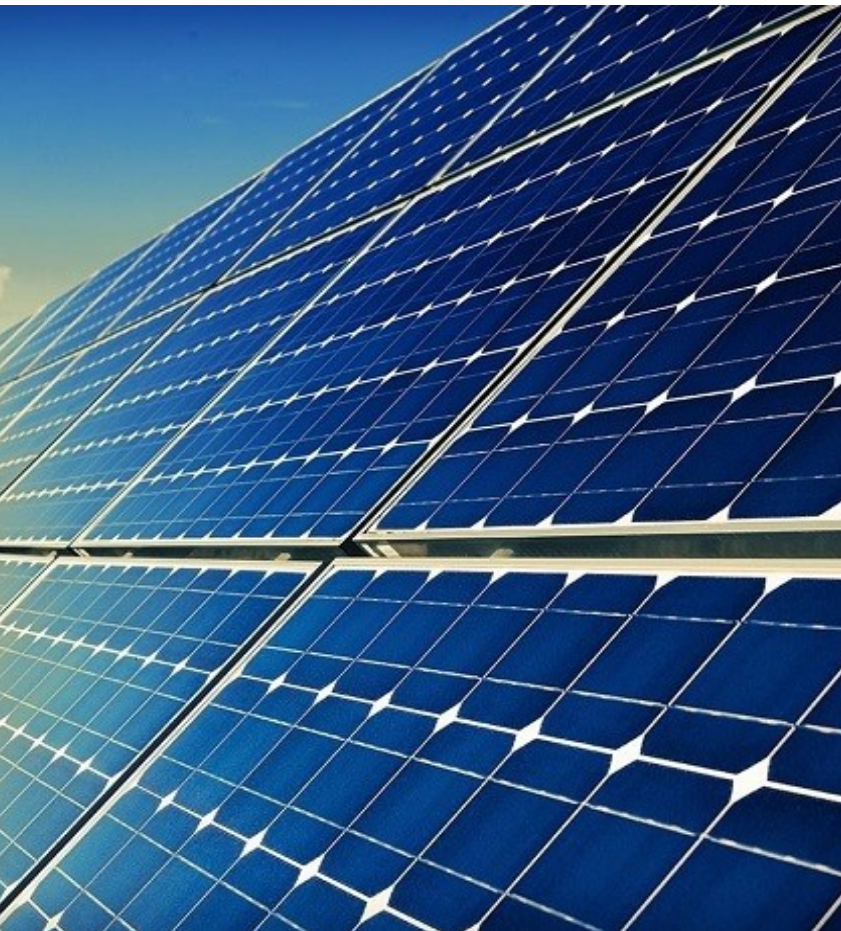
Solar power plant to inject electricity on the grid
